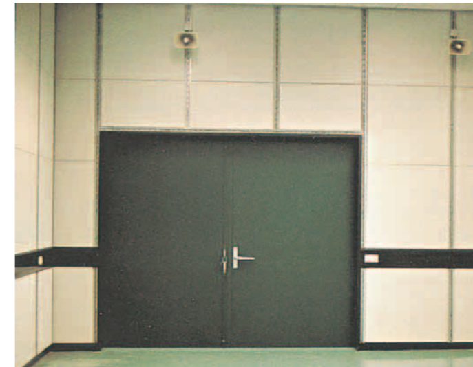
schalldämmendes 2-flügliges Tor, R_{WV} = 50\text{dB} sound retardant double-winged gate, R_{WV} = 50\text{dB}
